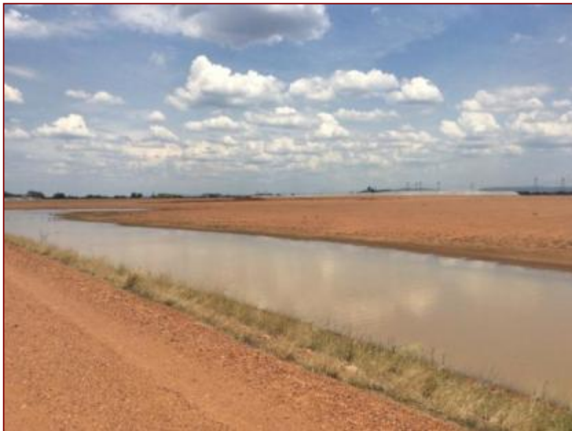
Figure 19 – The western end on the AFD
