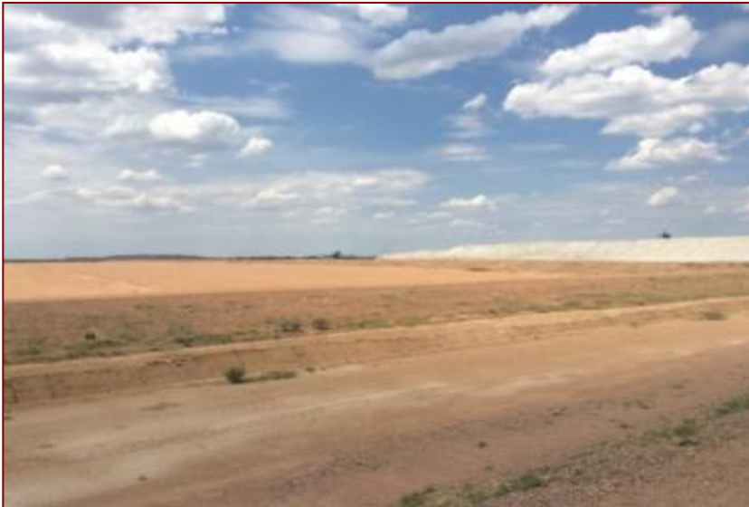
Figure 25- Image of the land dedicated to the facility and ash heap from Medupi power station. Taken from the south facing north-east
